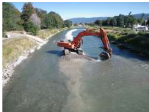
Construction of spawning gravel platforms in the Okanagan River in Penticton.
